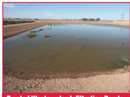
Treated Wastewater Infiltration Ponds
