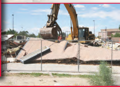
500 Building Demolition Completed December 8, 2014
