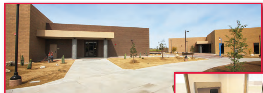
Career Technical Education Facility Completed May 1, 2014
