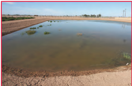
Treated Wastewater Infiltration Ponds Completed February 1, 2014
