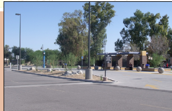
Bus Terminal Phase II
